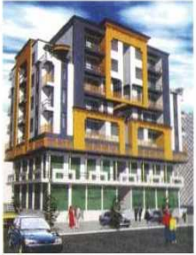
VINAYAK ENCLAVE Vaishali Nagar, Jaipur
